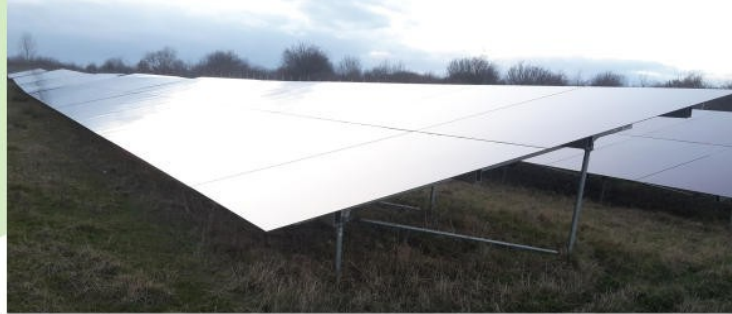
Monokristalline PV-FFA in Gotha, Foto: KGW
